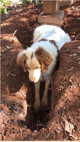
Angel digging deck footings by paw
